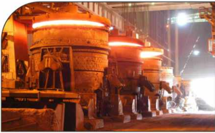
Iron & Steel Plant
