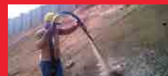
Concrete Spray on Embankment
