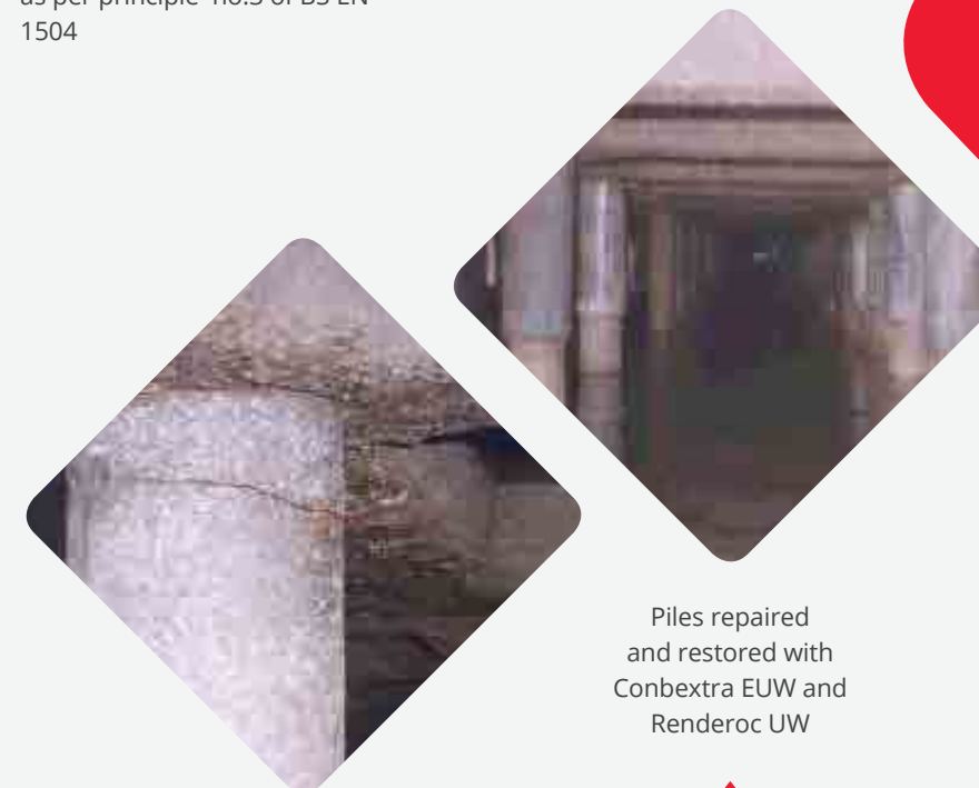
Cracks in the Jetty piles
