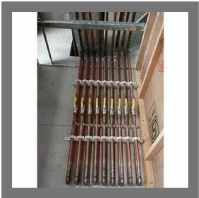
Medical Gas Pipe Line System
