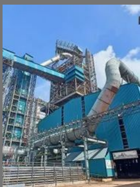
Industrial Roofing Services
