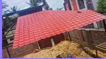
Color Coated Tile Roof work
